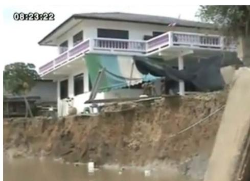
**Fig. 14.** Bank erosion by overloaded construction.
