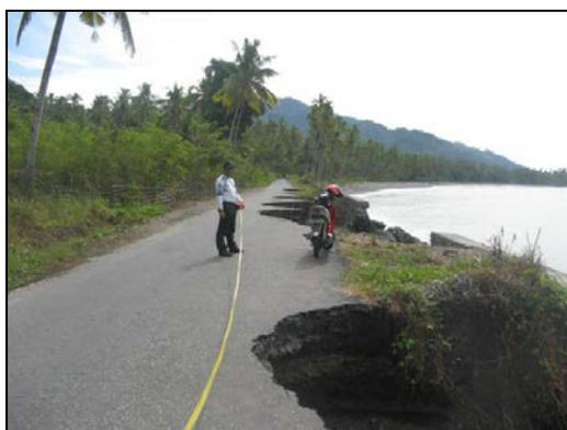
**Fig. 27.** Indication of creep along the road near to the shoreline
