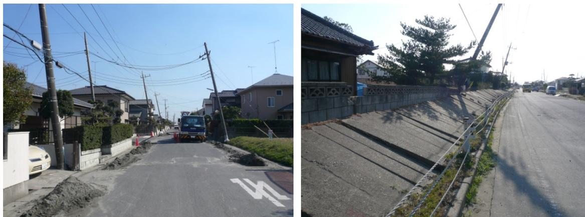
**Fig. 6.** Liquefaction-damaged district, Hinode, Itako City, including lateral spreading damage of a road (right).
