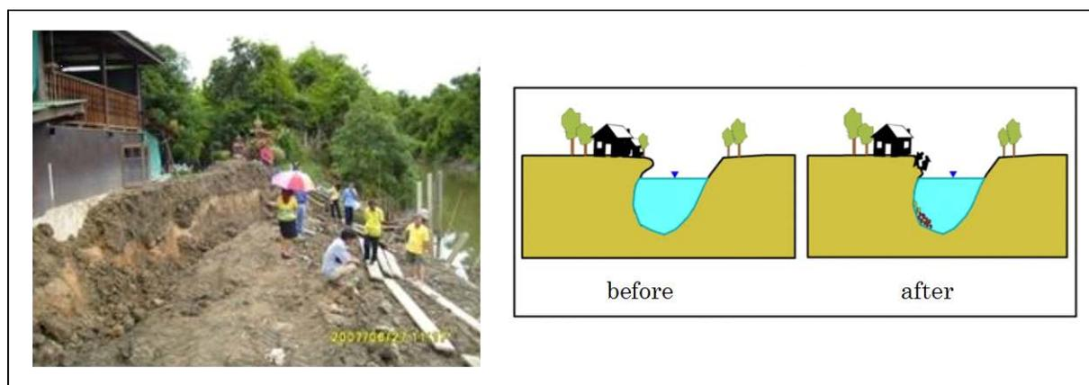
Fig. 7. Erosion in outer bank in Maeklong River.
