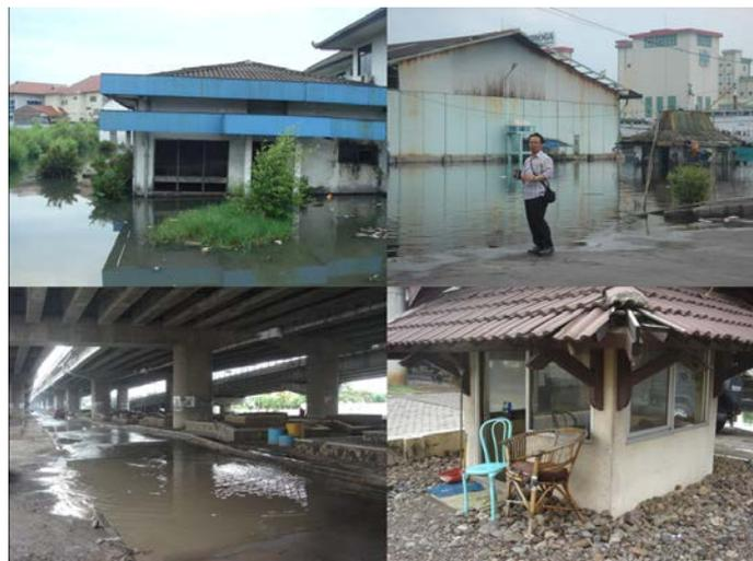
Fig. 22. The land subsidence in Semarang has caused damage to buildings, roads, railways tracks and other items of urban infrastructure.
