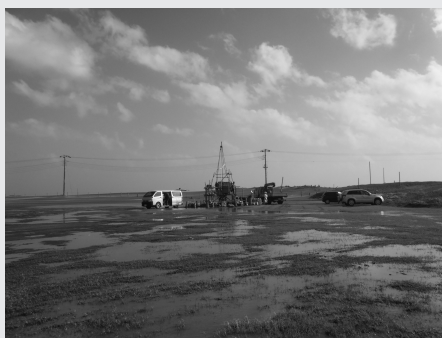
Boring survey in Kujukuri Plain, Chiba Prefecture.
