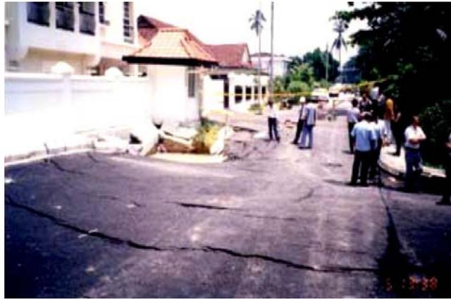
Figure 12: GESB sinkholes in 1995, possible cause of sinkholes due to nearby drilling and pilling works. (Source: Tang, S.M., 2005).
