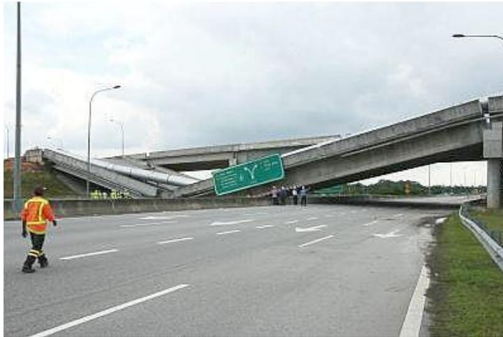
Figure 15: Recent overpass collapse in Cyberjaya Science Park. Construction was carried out in the alluvium cover of the Langat basin. (Source: The Star, Malaysia).
