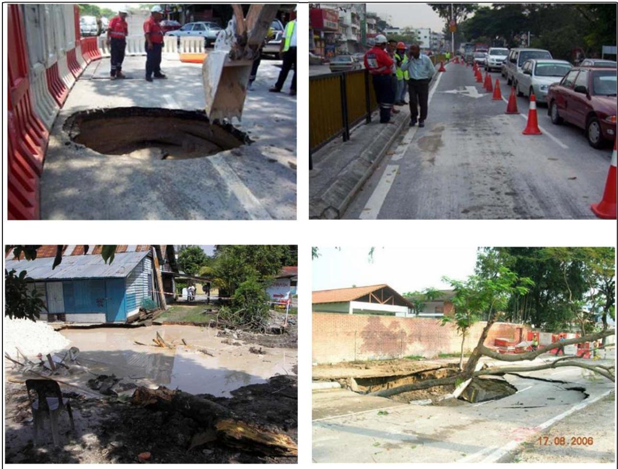
Figure 11: Numerous sinkholes and ground settlement occurrences within the Kuala Lumpur city limit during the construction of the SMART tunnel between 1998-2005. The events resulting substantial damage to properties and causing traffic disruption. (Photo from undated The Star news articles).
