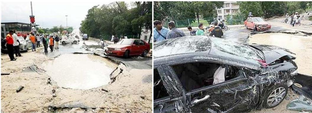
Figure 13: Sink holes developed in Jalan Universiti due to pipe burst destroying vehicles and injury to commuter. (Source: The Star Malaysia, 27/04/2010).
