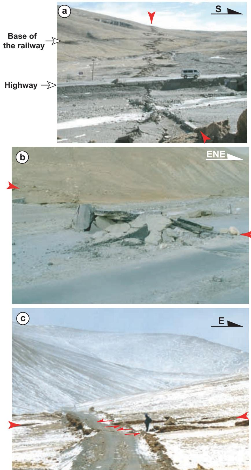
Fig. 11. Engineering damage of the highway and the base of Qinghai-Tibet railway across the rupture zone near the mile tablet of 2894 km. (a) Rupture zone passing through the highway and base of the railway. (b) Close-up of the displaced highway near the mile tablet of 2894 km. (c) Laterally displaced railway base under construction. Note the bookshelf effect of the blocks. Total lateral offset is about 3.3 m.
